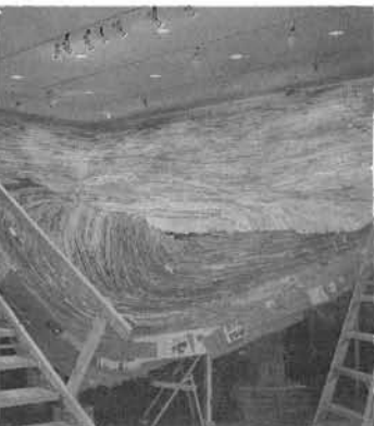
But you never forget that this is a construction site, propped up by all manner of silly structures.
